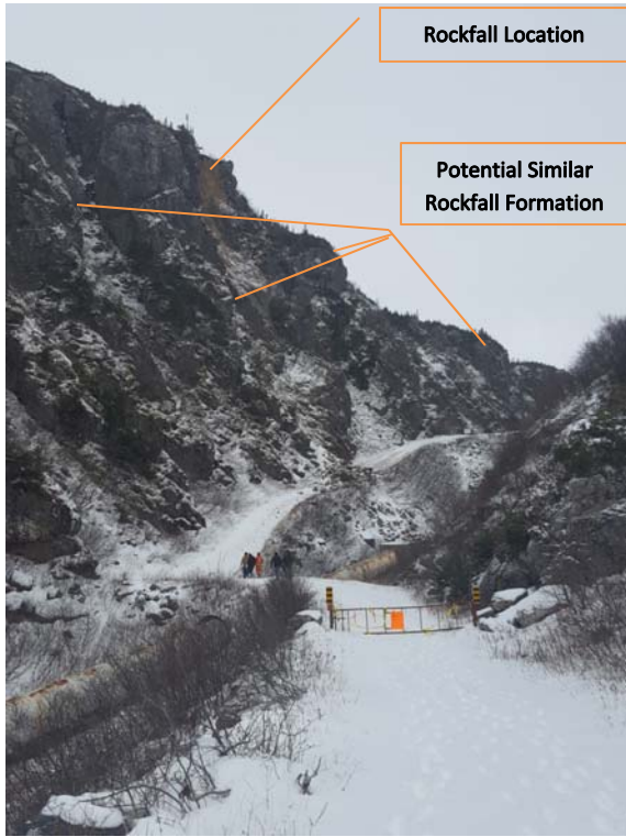
Photo 1 – View of the Rockfall Zone looking North.
