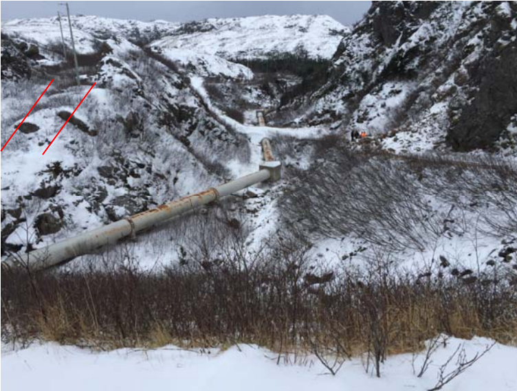
Photo 3 – Rockfall area looking south from the top of dam.
