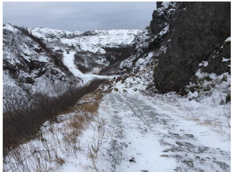
Photo 4 – Access road blocked by debris field.
